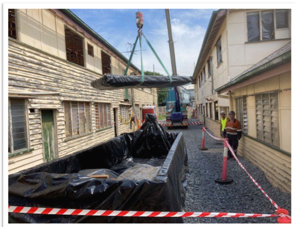
Figure 20. DOUBLE-WRAPPED PACKS BEING CRANED DOWN INTO LINED ASBESTOS WASTE SKIP.
