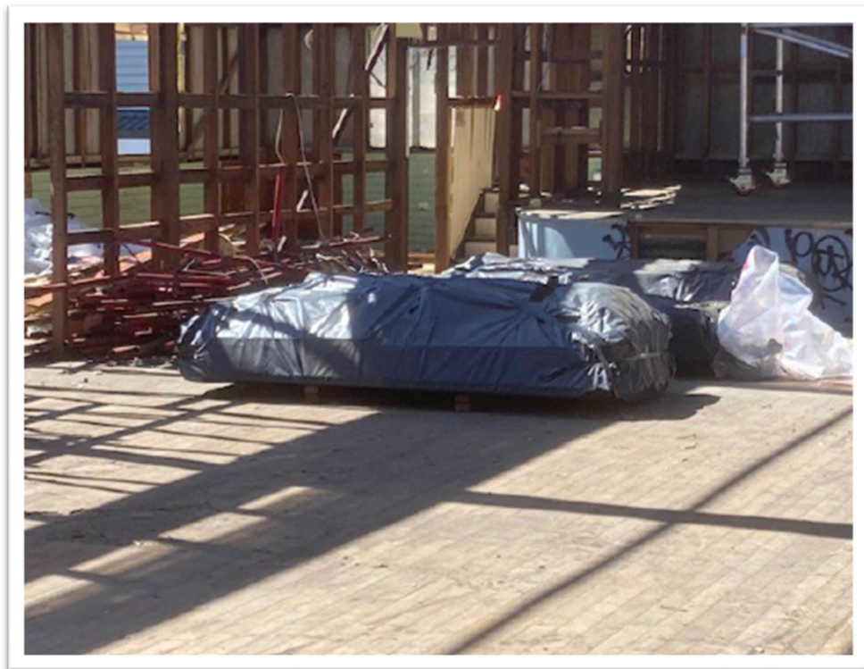
Figure 24. HANDLING AND ENCAPSULATION OF ACM SHEETING.
