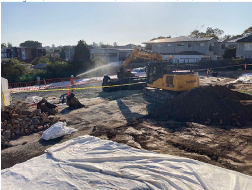
Figure 31. WATER SPRAY DUST SUPPRESSION OF SOIL BEING LOADED INTO SKIP
