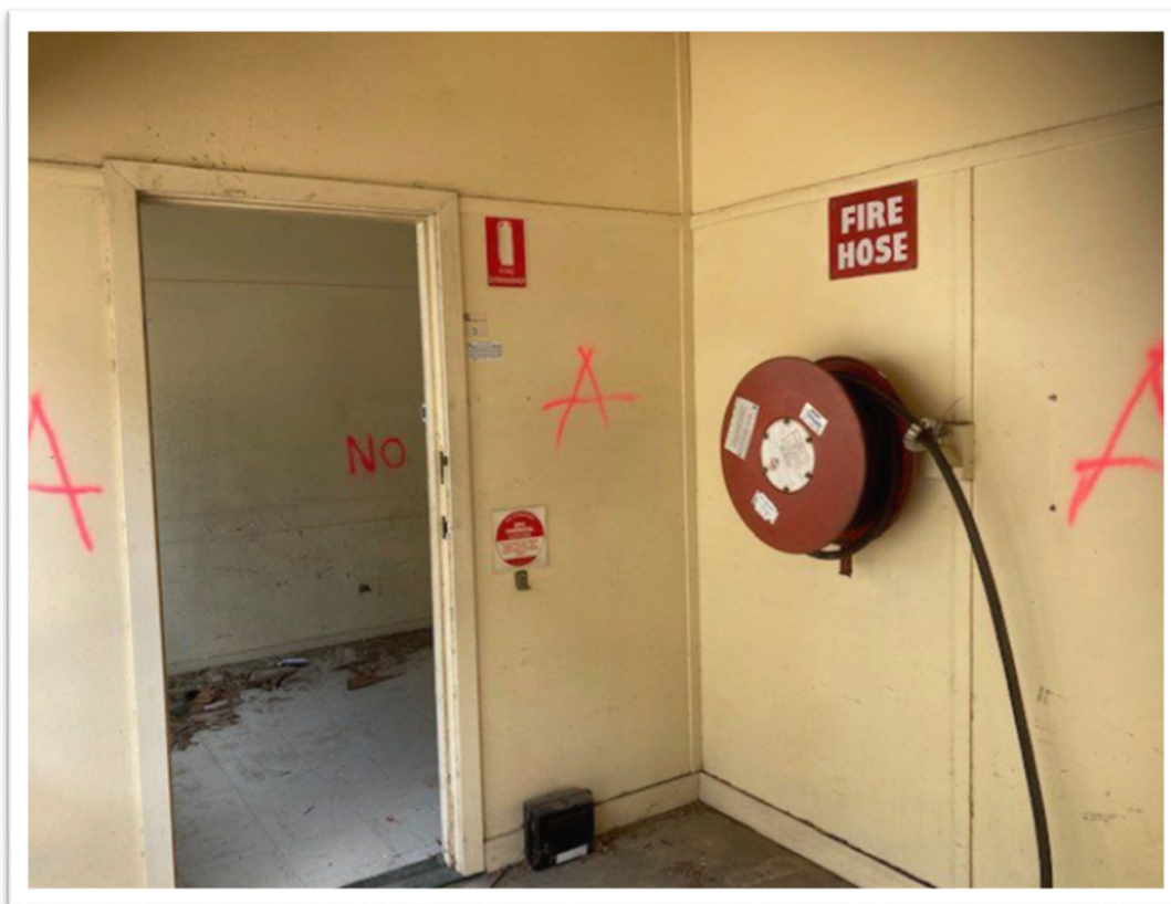
Figure 8. WALLS MARKED "A" FOR ASBESTOS OR "NO" FOR KNOWN NON-ASBESTOS
