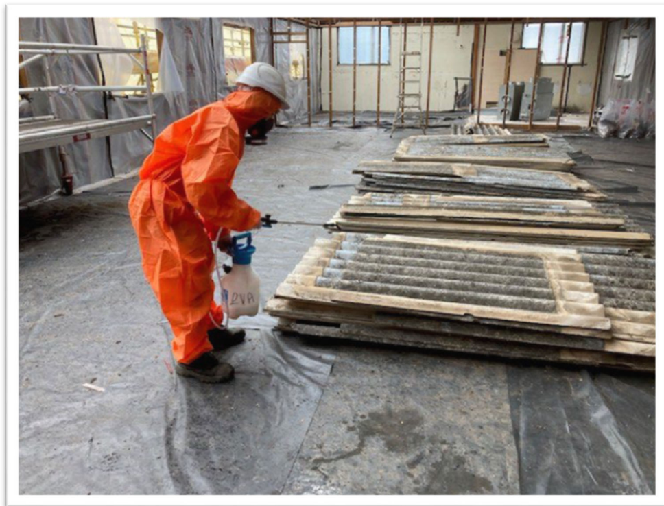
Figure 21. PVA SEALANT BEING APPLIED TO ACM SHEETING PRIOR TO HANDLING FOR LOAD OUT.
