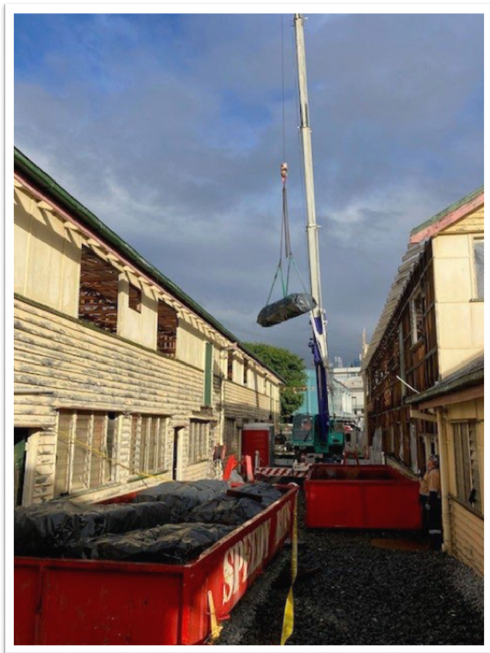
Figure 25. DOUBLE WRAPPED BUNDLES OF ASBESTOS WASTE BEING CRANED DOWN IN SOFT SLINGS
