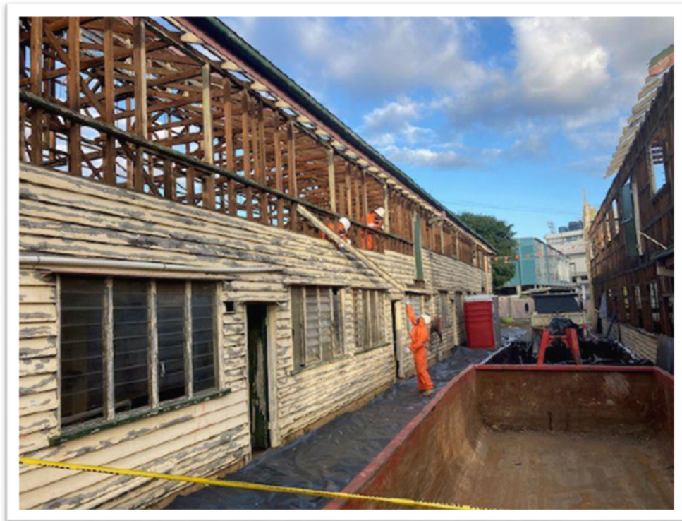
Figure 26. CONTROLLED REMOVAL OF THE EXTERNAL TIMBER (ACM PAINT)
