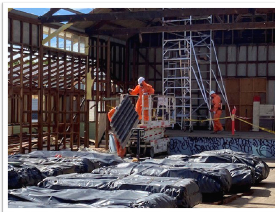
Figure 24. HANDLING AND ENCAPSULATION OF ACM SHEETING.
