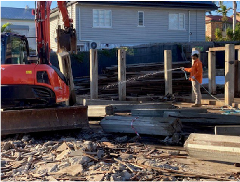
Figure 32. WATER SUPPRESSION DURING MECHANICAL DEMOLITION
