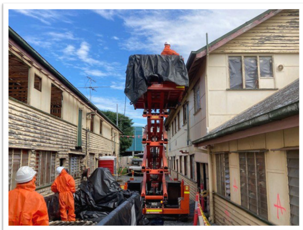
Figure 22. EWP (SCISSOR LIFT) BEING USED TO LOWER ACM SHEETING FOR TRANSFER TO WASTE SKIP
