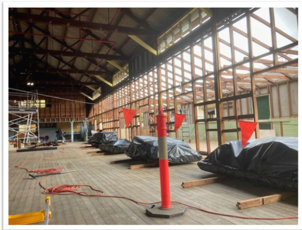
Figure 19. VARIOUS ENCAPSULATED PACKS READY FOR CRANING
