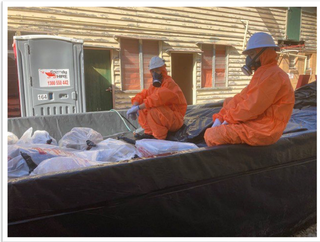
Figure 12. ASBESTOS REMOVAL CREW MEMBERS READY TO RECEIVE DOUBLE WRAPPED ASBESTOS WASTE FOR CAREFUL PLACEMENT IN WASTE SKIP
